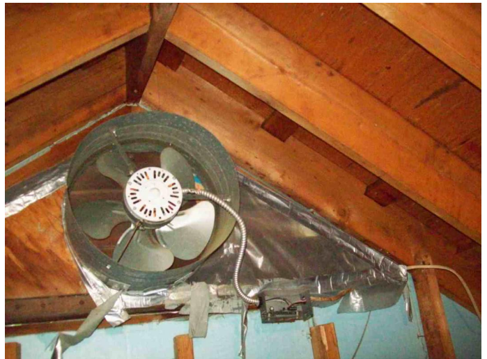
Remove gable end vent fans.
